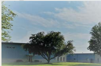
OILGEAR FREMONT, NE USA
